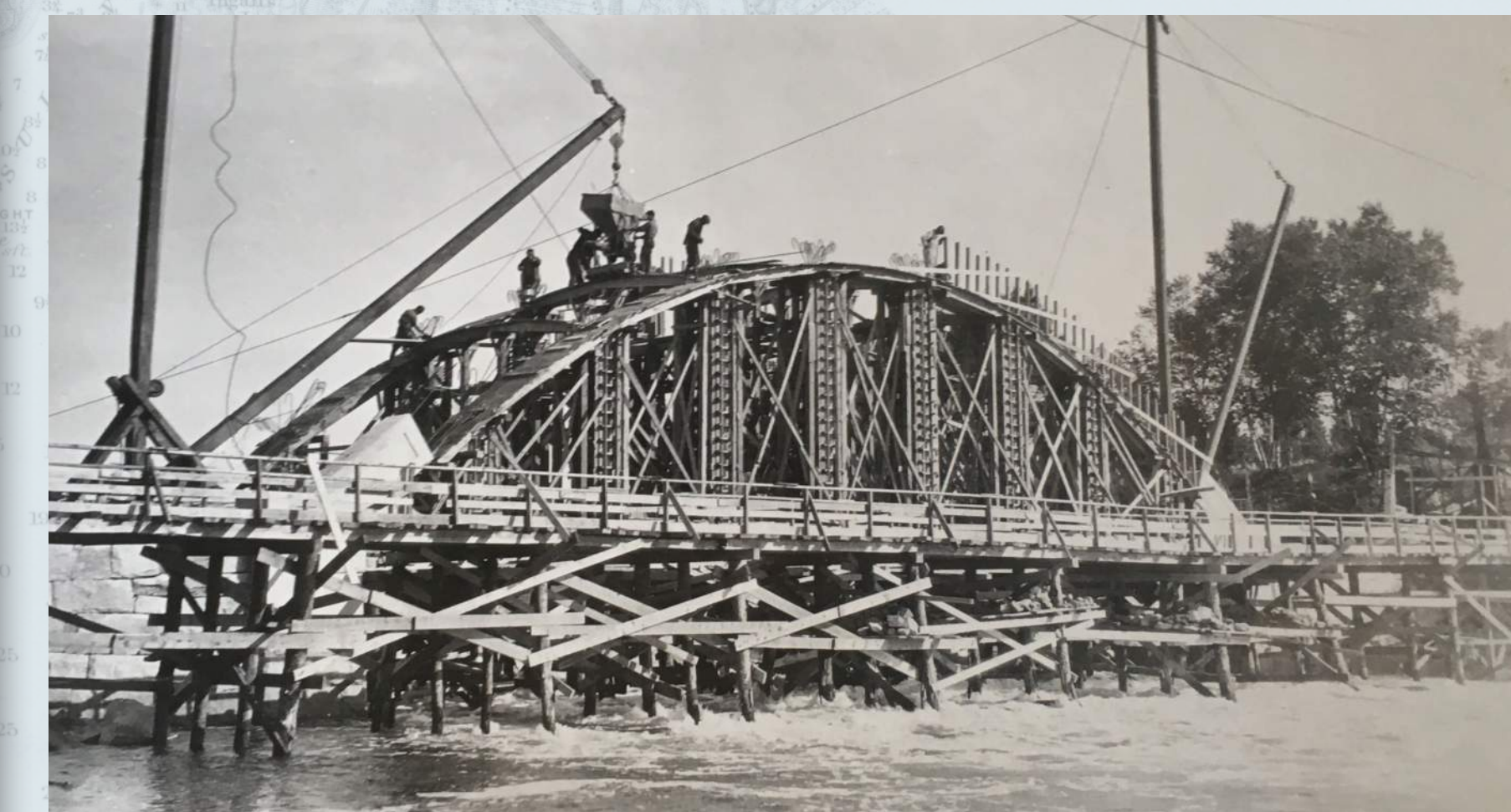
The 1926 tied arch bridge under construction (courtesy Maine DOT).
